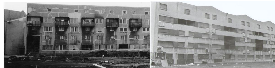
Picture – Before WGHC: Deck access flats in West Granton prior to demolition in 1993.
